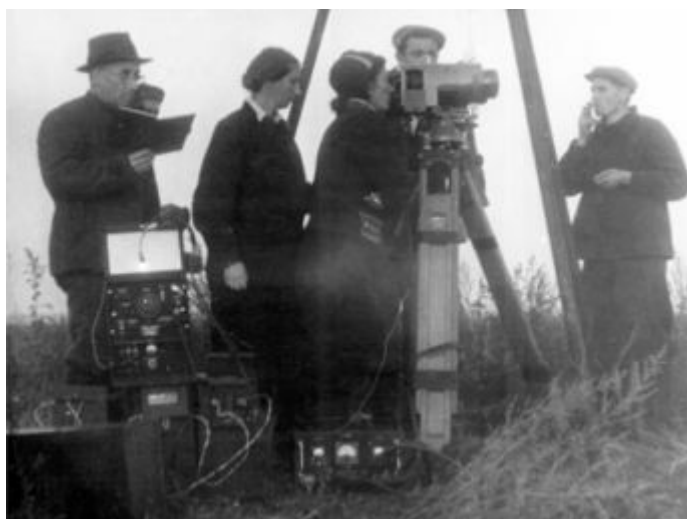
1953 Electronic distance meter SVV-1
