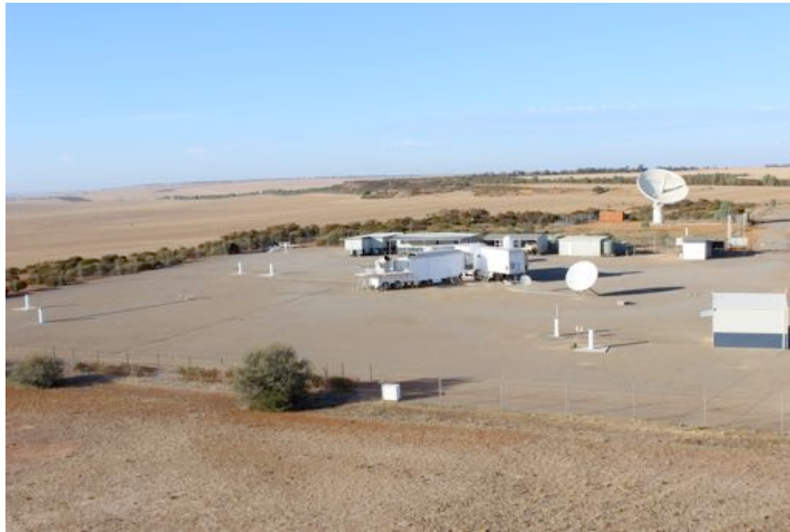
Figure 1.3: Yarragadee fundamental geodetic observatory, with GNSS in left of image, SLR station centre, and VLBI antenna rear-right of image
