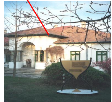
Caldarusani Geodynamic Observatory
